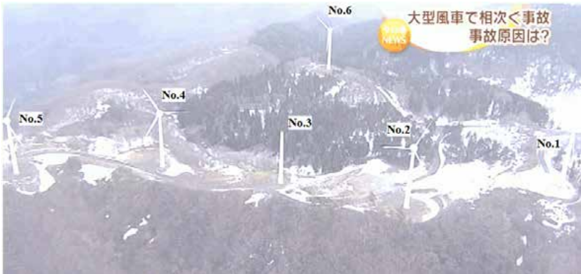
Fig.2 Picture of wind turbine accident, quoted from RKB Mainichi Broadcasting Corporation
